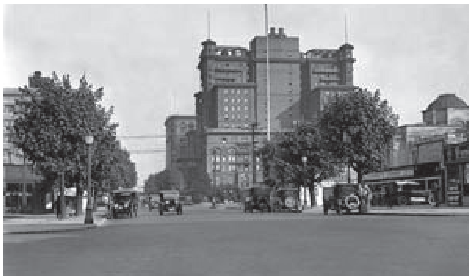
LEFT: The city's second Hotel Vancouver at Granville and Georgia, seen from Georgia at Burrard.
