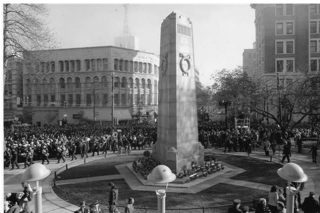
BELOW: Victory Square, November 2003.
